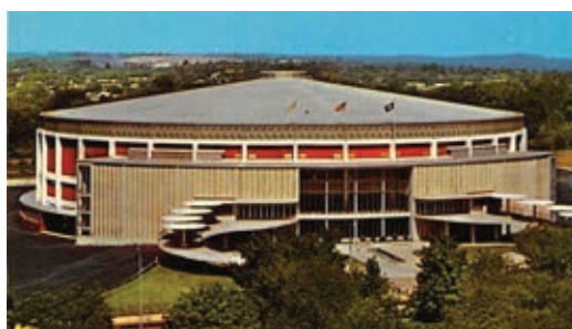
E. A. Diddle Arena Photo above from the Internet
